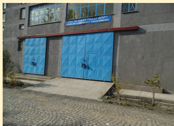
Ramp constructed to enable access to classrooms and workshops
