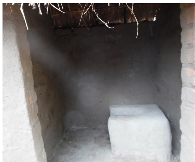
Accessible Pit Latrine
